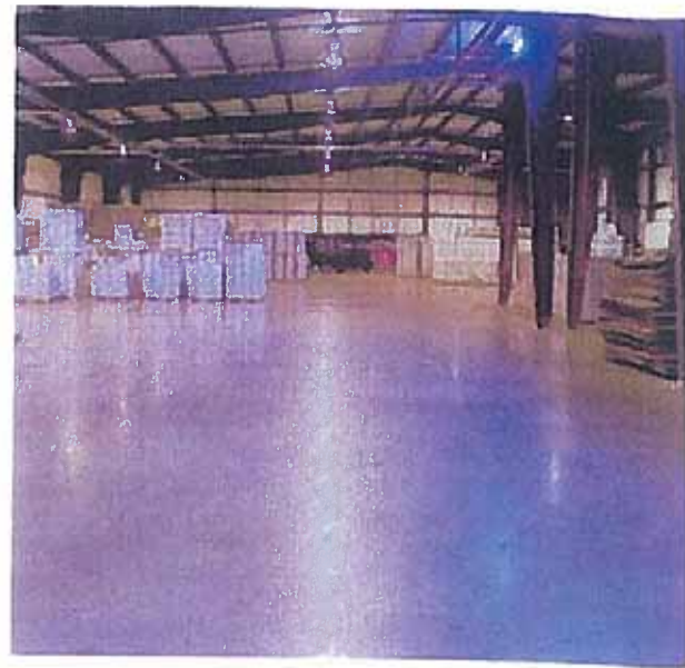
A 127x60 foot warehouse floor slab 6 inches thick with HVSF and no joints or cracks after three and a half years.
