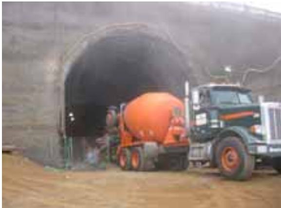
FORTA-FERRO®-reinforced tunnel lining for Clo de la Tech Winery in California
