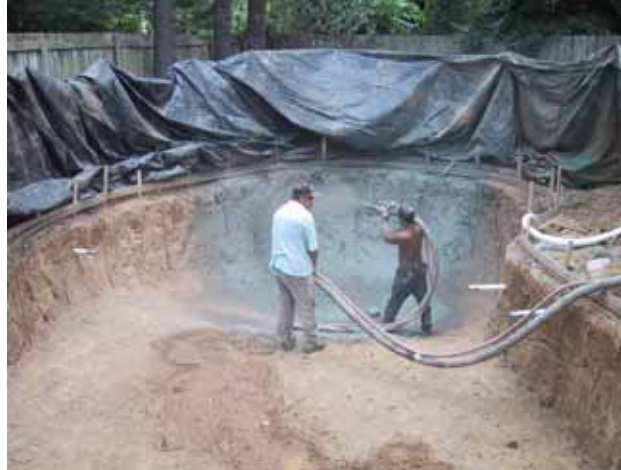
FORTA-FERRO® reinforced swimming pool – Germantown, TN
